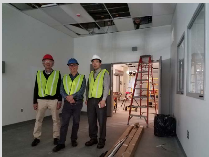
FIS cabin under construction
